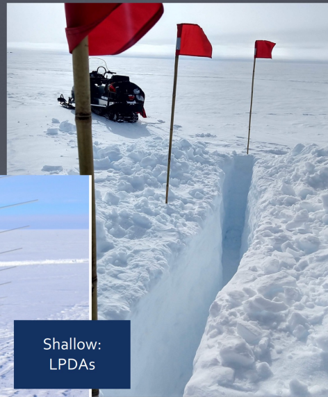
Shallow antennas deployed in trenches
